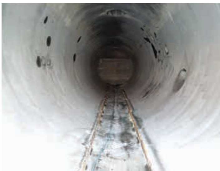
Figure 4: In July 2015, after four years in service, the reboiler was again opened up for inspection. No further pitting damage or corrosion was identified.
