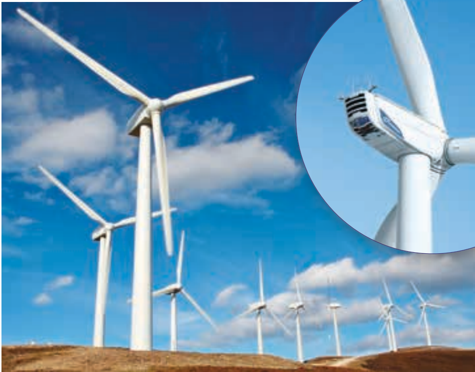
Above: The Amakhala Emoyeni project involved the installation of 56 Nordex 2.4 MW N117 wind turbines specially developed for low-wind sites.
