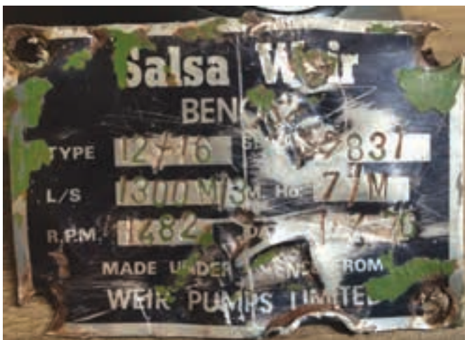
The original Salsa Weir product information plate from a Uniglide pump installed in 1976.
