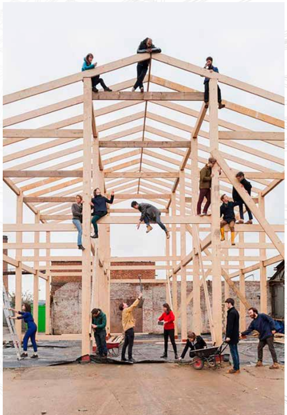
Building the studio
