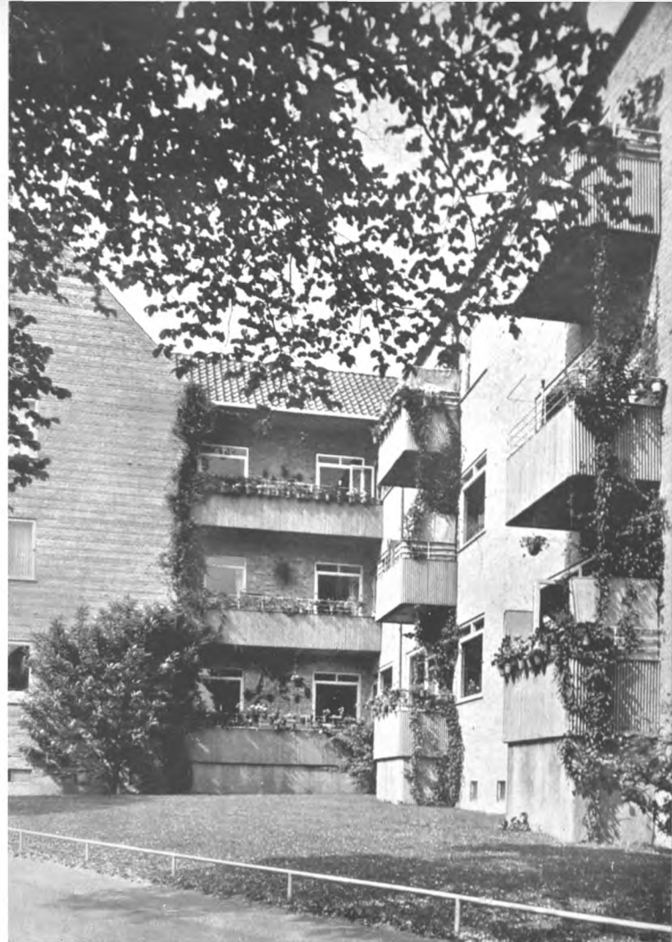
South-west corner facing Tagensvej.
