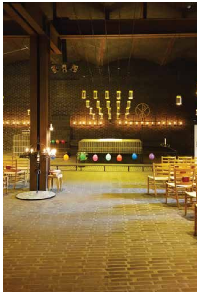
ABOVE AND BELOW: St Mark's brick vaults supported on angled steel beams. (All Images: T. Deckler.)
