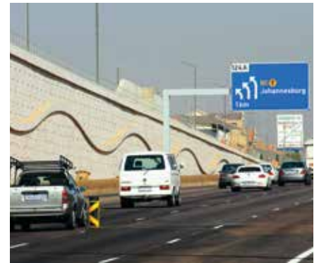
John Vorster offramp to Viaduct 5.
