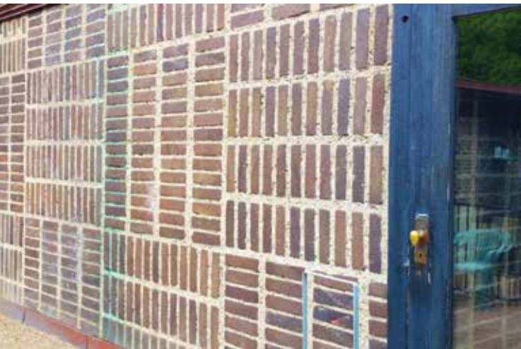
Exterior of vestry offices at Sankt Petri showing various brick patterns.
