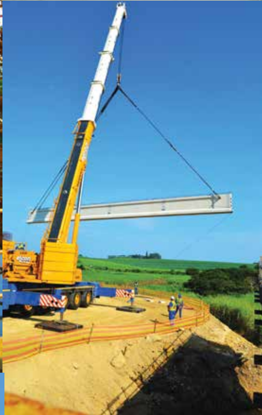
TOP LEFT: A post tensioned beam being manoeuvred into position at Mlalazi River bridge.
