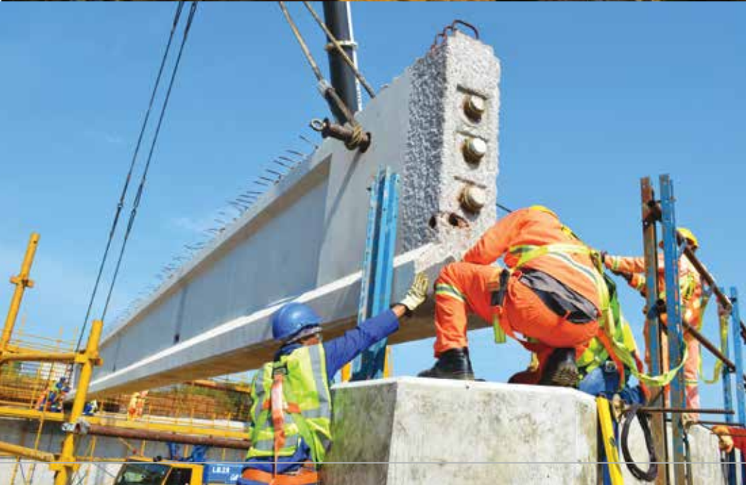
TOP LEFT: A post tensioned beam being manoeuvred into position at Mlalazi River bridge.
