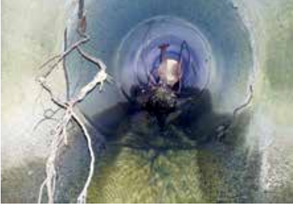
Pipeline before CIPP installation.
