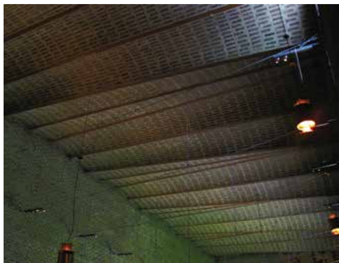
ABOVE AND BELOW: St Mark's brick vaults supported on angled steel beams. (All Images: T. Deckler.)
