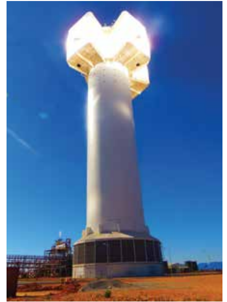
ABOVE: !Khi Solar One Tower at Upington, Northern Cape, clearly showing how concentrated solar power (CSP) systems concentrate the sun's energy using the reflection from the mirror panels to produce heat that is then used to generate electricity.
