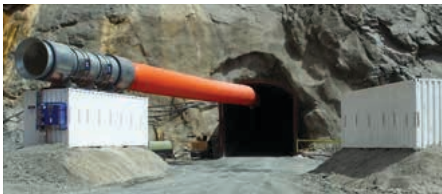
The 1200 portal at the Syama underground mine (photo: Resolute).
