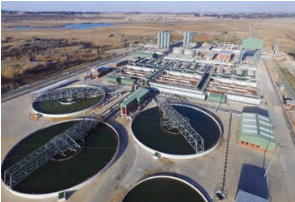
View of the completed Eastern Basin Acid Mine Drainage (AMD) treatment plant.
