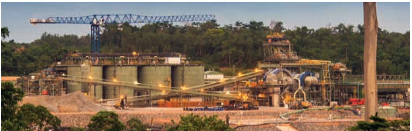
The Asanko processing plant operated at an annualised rate of 3,6 Mt/a (20 % above design) during Q4 following crushing circuit upgrades in late Q3 2016 (photo: Asanko Gold).
