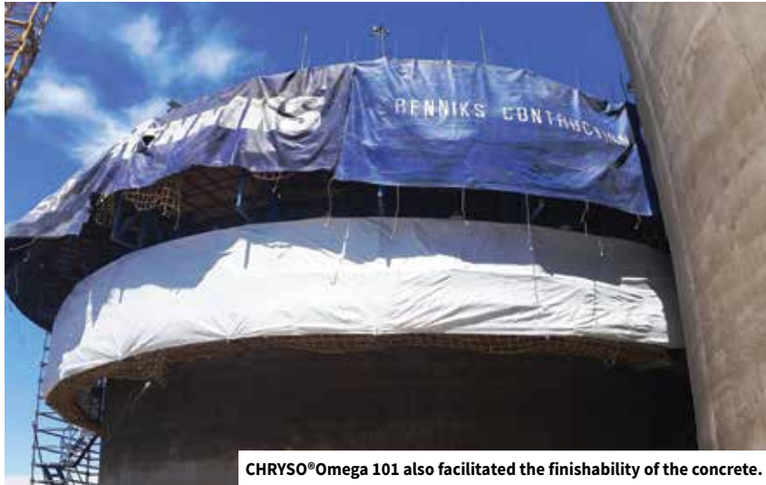
CHRYSO®Quad 20 increases the cohesiveness of the concrete and prevents bleeding and segregation, improves the finishability of the concrete and assists construction by giving the concrete its sliding effect.
