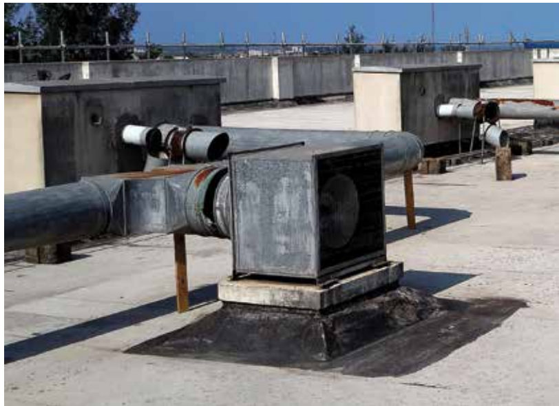
a.b.e. Construction Chemicals supplied its unigum torch-on bitumen membrane for the waterproofing of Maputo's Universidade Eduardo Mondlane.
