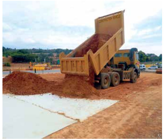
Base layerworks being constructed over the reinforcing RockGrid PC layer.
