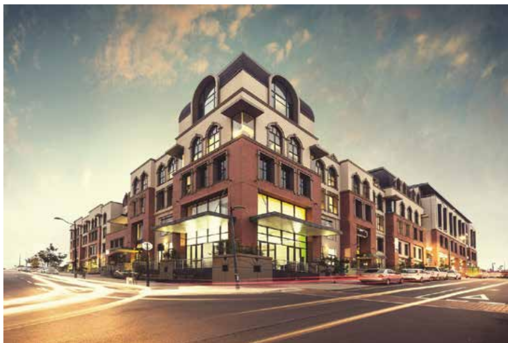
Growthpoint currently owns or co-owns the largest portfolio of Green Star SA certified buildings of any company in South Africa, with 23 buildings rated so far.
