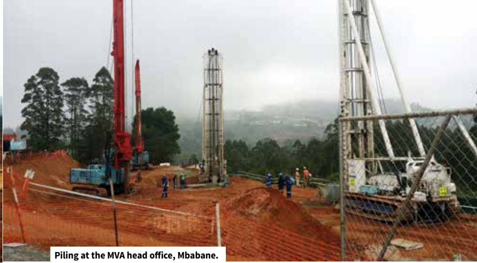
Piling at the MVA head office, Mbabane.
