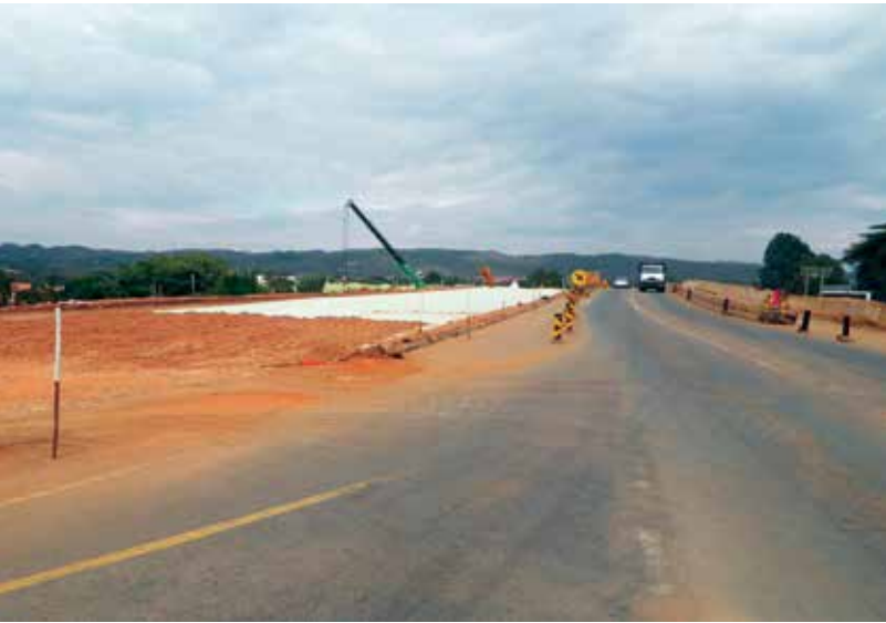
Additional lanes were created on Simon Vermooten Road.
