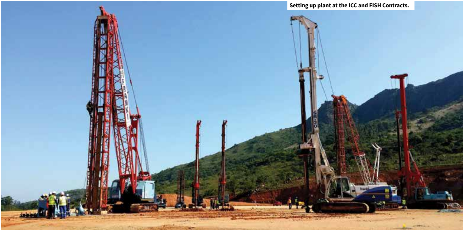
Setting up plant at the ICC and FISH Contracts.
