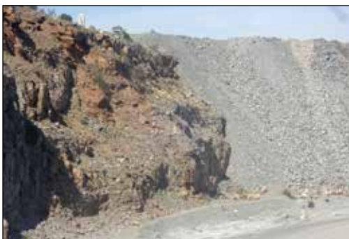
Figure 1: Sandy rock trap designed to stop the rolling rock threat from above and act as a barricade and even a monitoring device, if rock is trapped.
