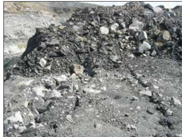
Figure 5: A mine with safety berm placed on a crest edge that covers the prominent tension cracks. It is so high that a person would have to stand on the loose material to see inside the void.
