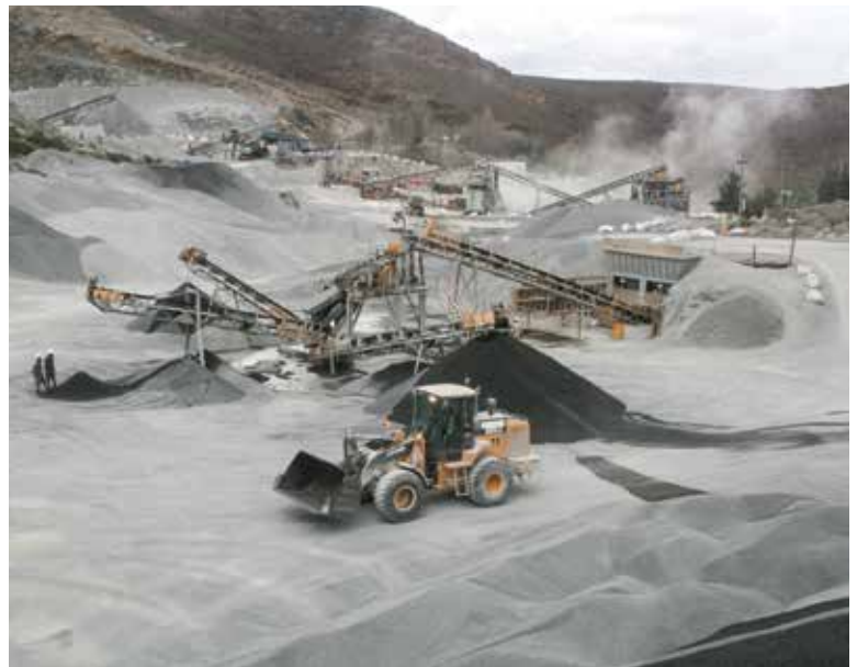
Second wash plant in the foreground. While taking the photograph, the plant had just been started up, hence the dust in the background.
