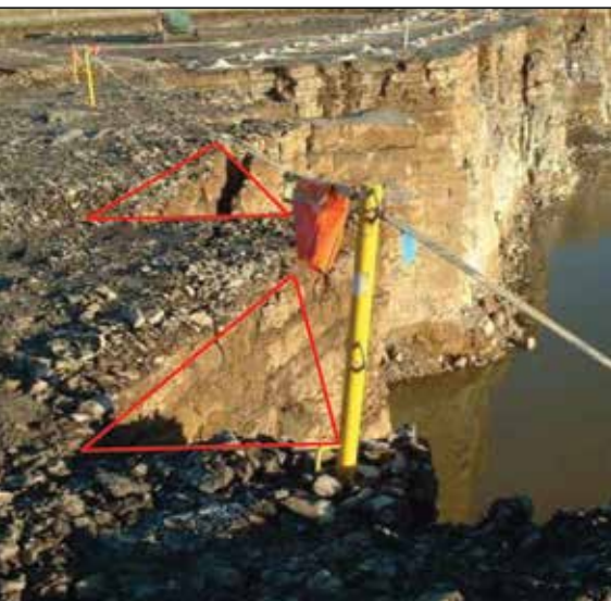
Figure 9: Photograph of a UK quarry with well-constructed but poorly-positioned barrier (Source: QNJAC).
