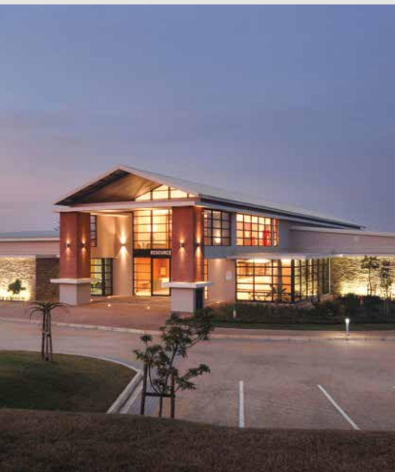
BEKA Schröder supplied an holistic exterior and interior lighting solution.
