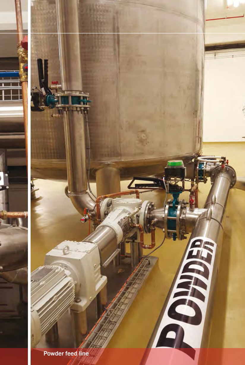
Tank bottom valve and manual shut-off valve, both with electrical position indicator LSR
