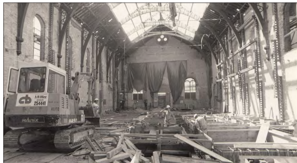
Work is carried out to completely refurbish the Corn Exchange in 1992
