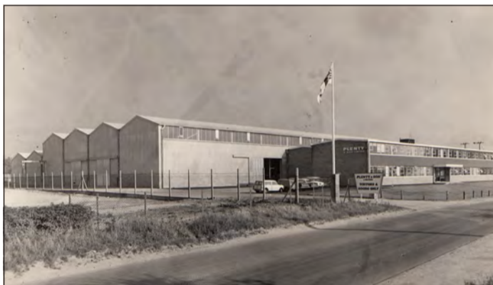
Plenty & Co's New Eagle Iron Works which opened in Hambridge Road in 1965
