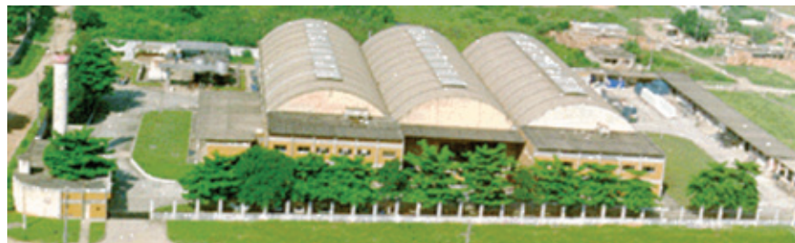
○ The Agena plant in Brazil
