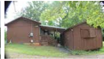
850932 - ANNA BRYANT TRL - Wood floors and other materials were cut from the surrounding land. House has open kitchen, living area, dining area 1.5 BA, 2 BR and a detached screened in porch with storage on one end. HVAC system consist of individual Global Ductless Air Conditioner units in various locations throughout the house for a nice even heating and cooling. $82,100
