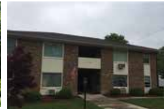
835202 - 1707 N MAIN ST - CONDO - Brand new heat pump & painting throughout! Great value for the money! 2 bed, 2 bath condominium with many closets! HW floors throughout, new windows, large living room. Make your appointment today! $84,500
