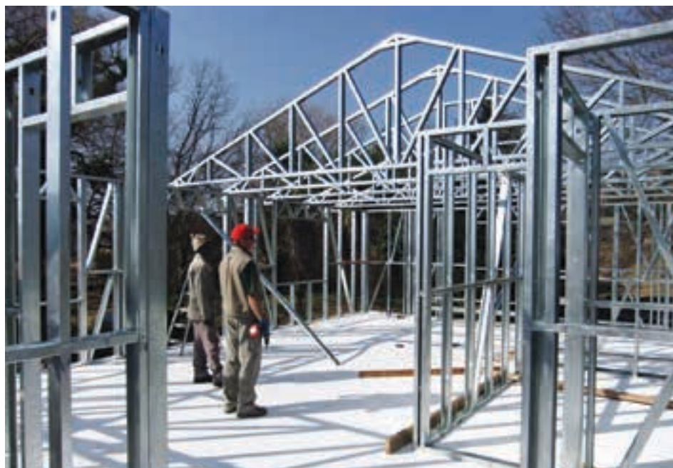
A growing number of architects, materials manufacturers and builders are embracing new construction technologies such as light steel frame building.
