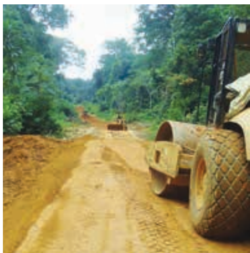
An access road under construction at the Dugbe project.
