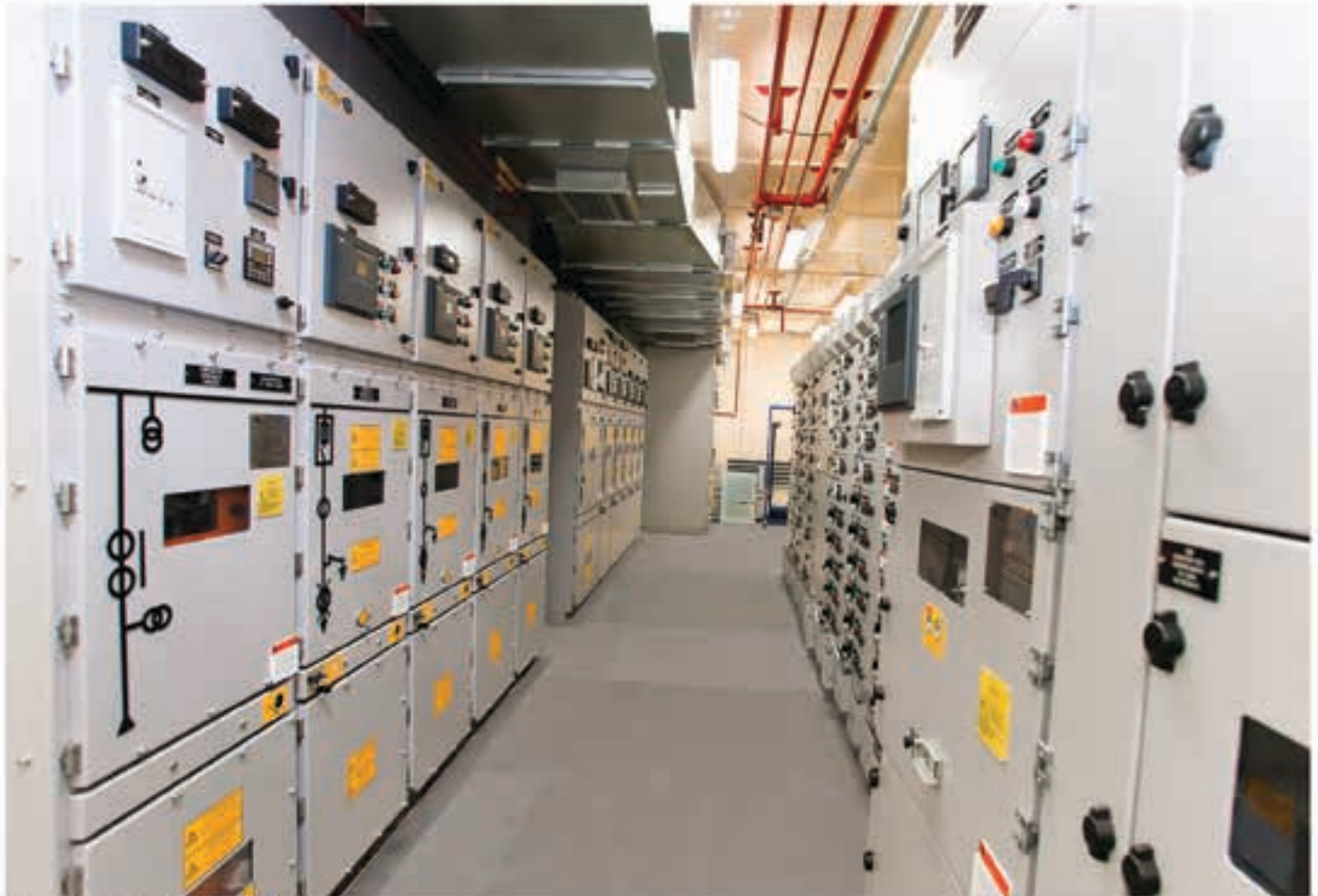
LV and MV Switchboards inside "E" House
