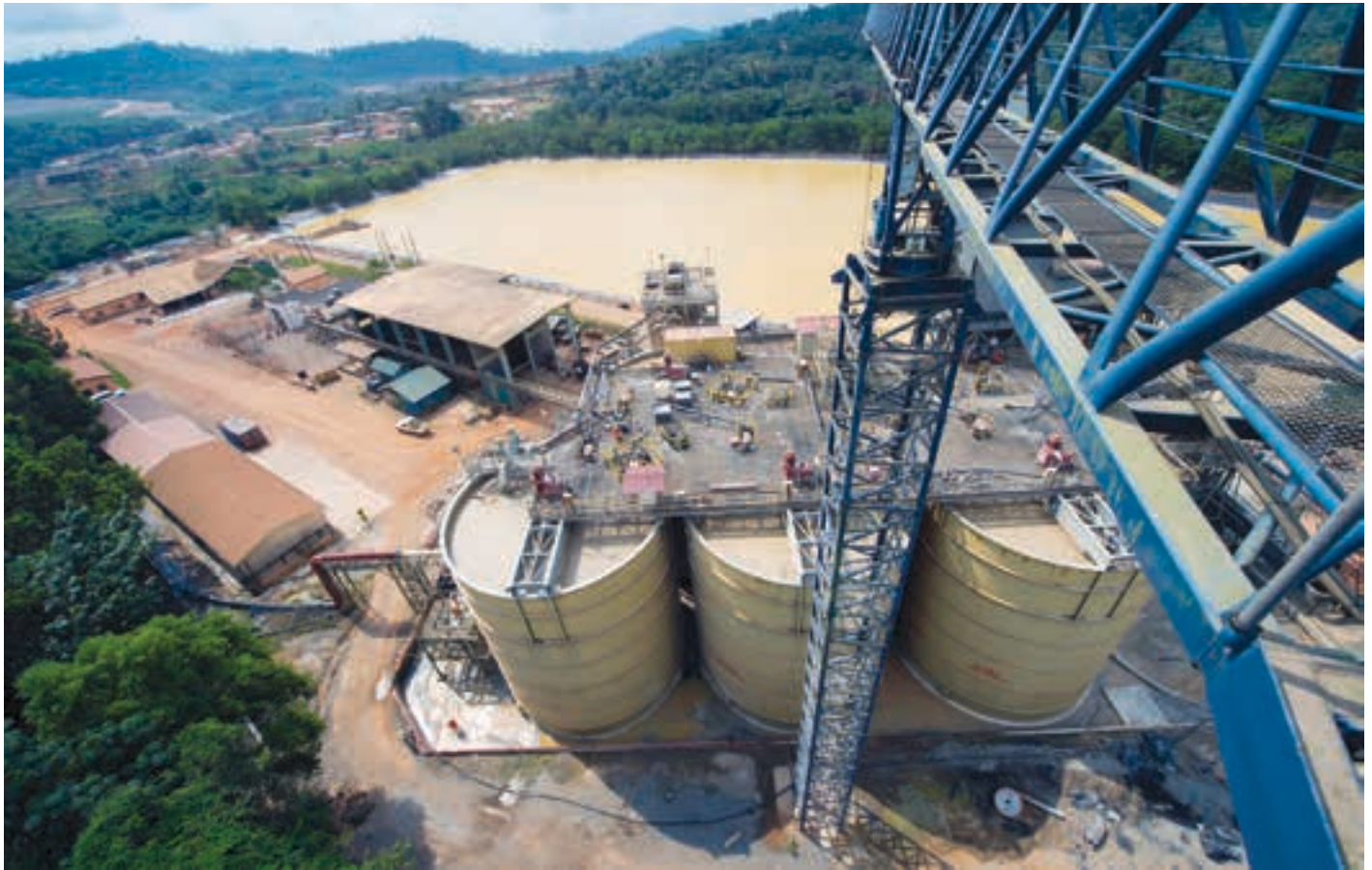
Wassa has a carbon-in-leach processing plant with a rated capacity of 2,7 Mt/a (photo: GSR).
