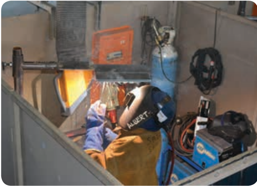
A trainee producing fillet welds on plate in the 4F (overhead) position.
