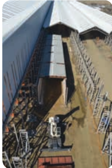
Below: In addition to the new Bay 4 and its machine shop (left), Bays 1 to 3 at Sky Hill are also being extended to the full 500 m length, with the heat-treatment furnace being moved and upsized to 15x15x80 m.
