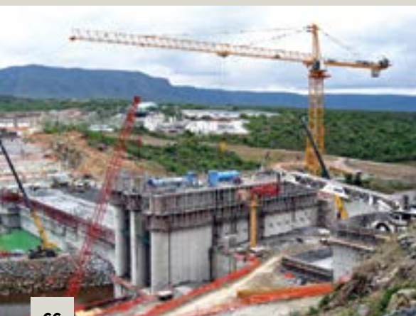
A Potain tower crane played an important materials handling role in the construction of De Hoop Dam.
