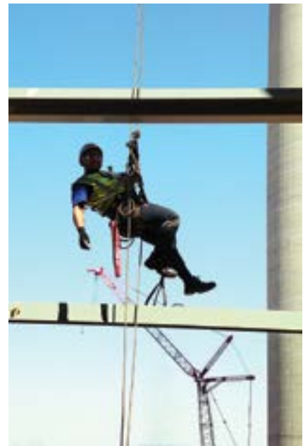
Workers operating high above ground.
