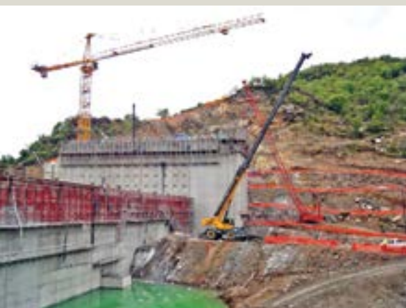
A Potain tower crane played an important materials handling role in the construction of De Hoop Dam.
