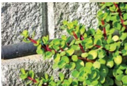
A pipe runs along each row, dripping water into each block.
