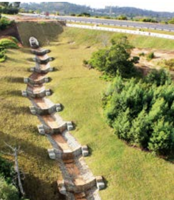
Hydraulic structures, gabions and mattresses (Hornlee, Western Cape).
