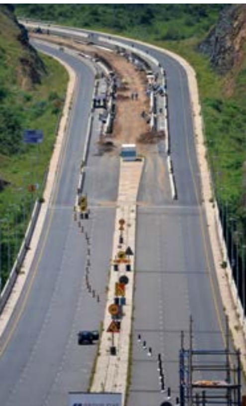
Construction of the dedicated Bus Rapid Transit lane on the MR577 (Provincial road) looking east from the bridge over the Umgeni River.
