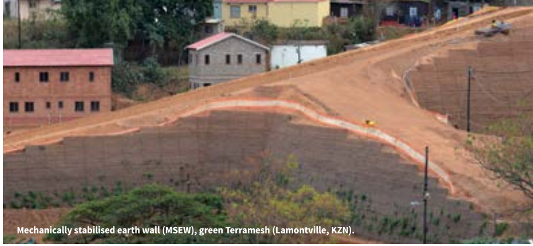
Mechanically stabilised earth wall (MSEW), Terramesh, Green Terramesh and Paraproducts (Hazyview slip repair on road D1043, Mpumalanga).
