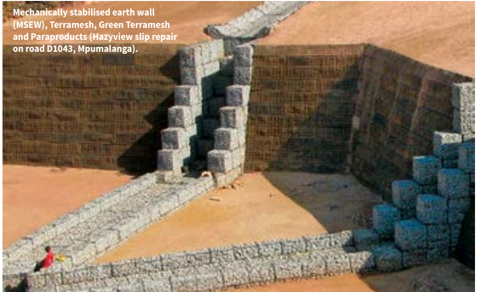
Mechanically stabilised earth wall (MSEW), green Terramesh (Lamontville, KZN).
