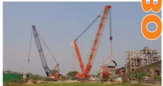
crawler cranes and heavy lift projects
