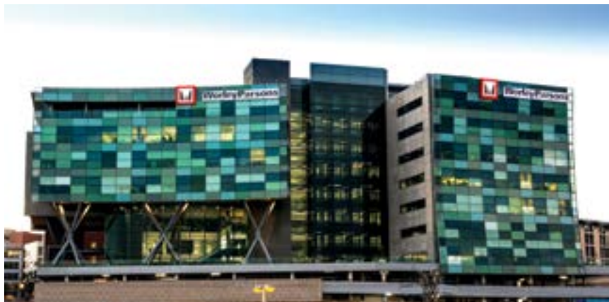
The WorleyParsons head office building in Melrose Arch, which was awarded a 4-Star Green Star SA Office v1 Design rating by the Green Building Council of South Africa.
