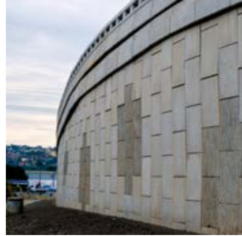
Mechanically stabilised earth wall (MSEW), MacRes (Umgeni interchange, KZN).
