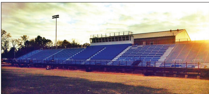
Bremen High School Stadium Renovation
