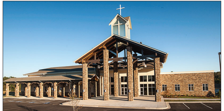
Roopville Road Baptist Church Addition
