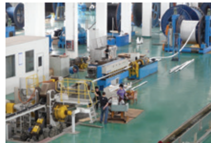
▲ A BWE SheathEx production line
