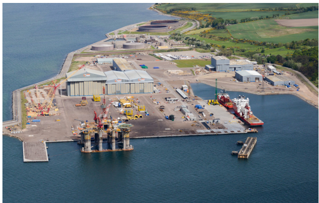
NEP Fabrication, Assembly and Load-Out
