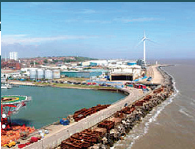
Hamilton Dock North
