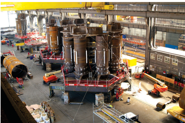
Pile Sleeve Clusters Fabricated for Kvaerner Verdal AS
