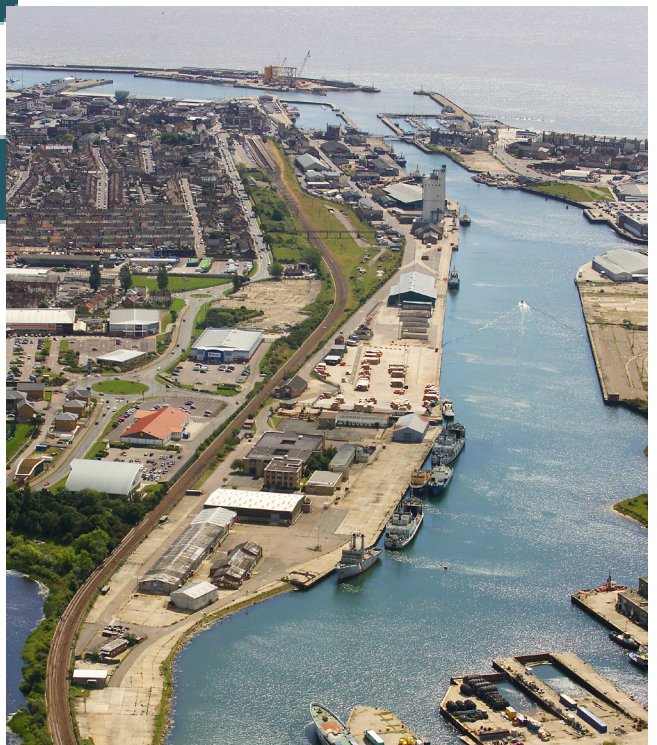
OGN Lowestoft Facility
