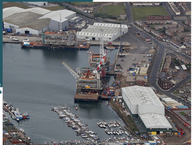
Heerema North Gate Facility
