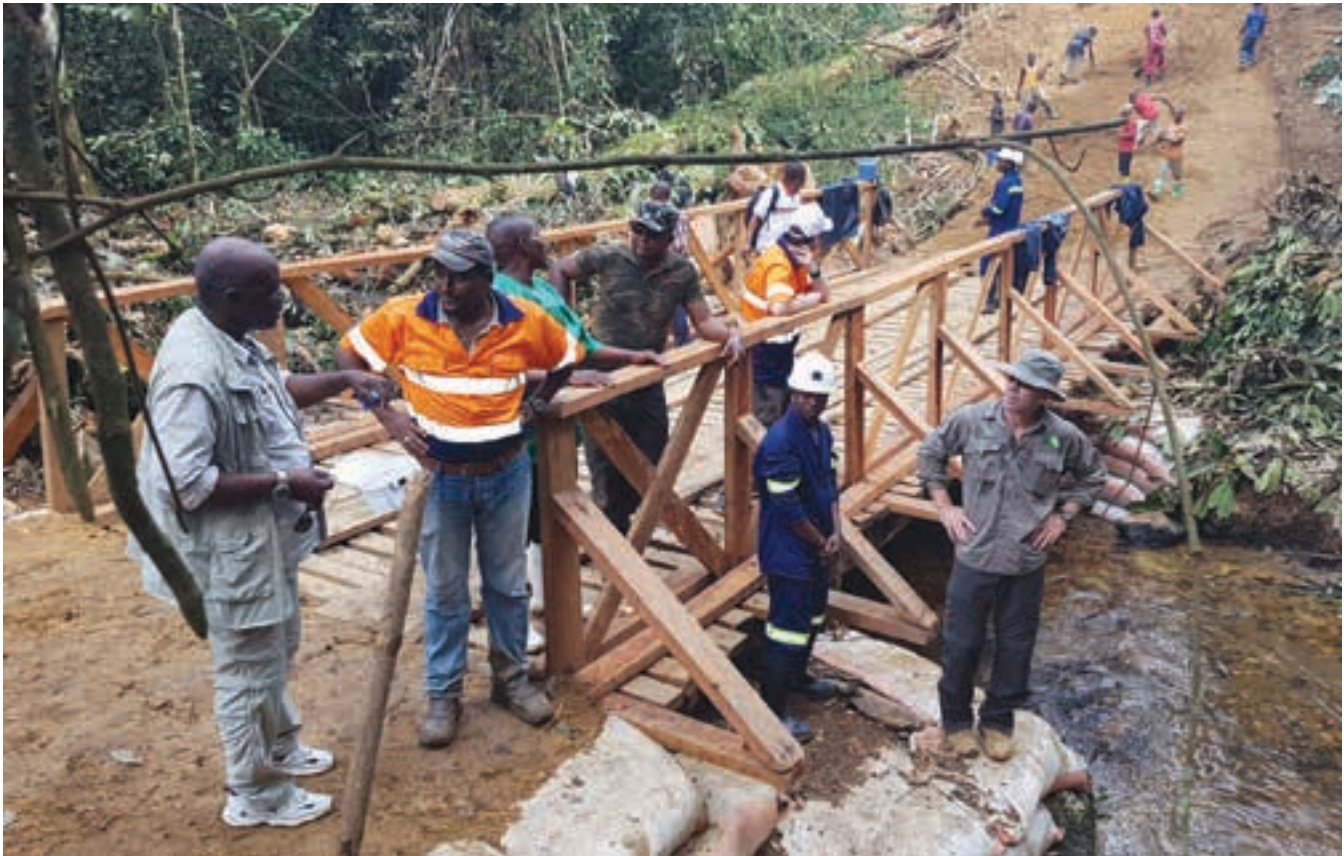
Alphamin team members at the Logu Bridge.
