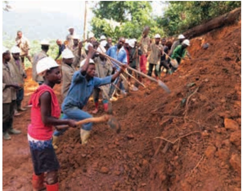
Drill pad preparation at Bisie using local labour.
