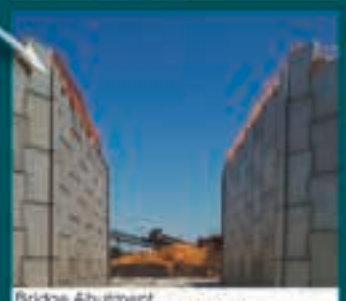
Bridge Abutment MACRES® T & PARAWEB® Black Rock Mine, Northern Cape
