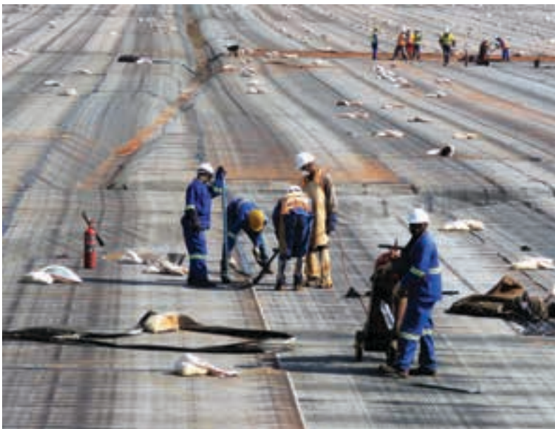
The TSF with welding of the liner seams in progress.
