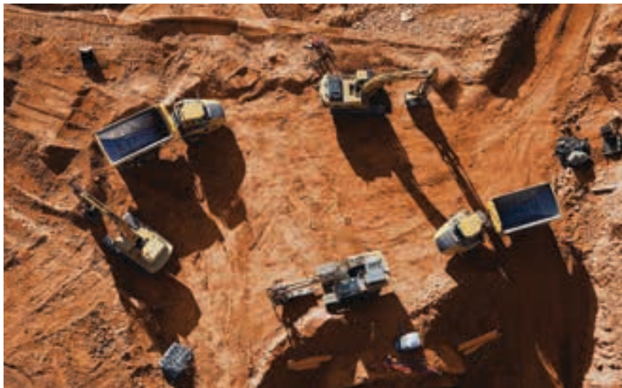
Articulated haulers and excavators at work at Yanfolila (photo: Hummingbird).
