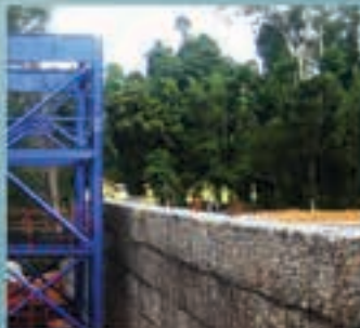
Mechanically Stabilised Earth Wall TERRAMESH® & PARAGRID® Liberty Mine, Liberia
