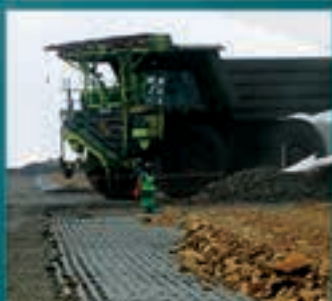
Basal Reinforcement - PARALINK® Grootegeluk, Limpopo
