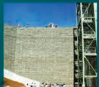
Mechanically Stabilised Earth Wall TERRAMESH® - Marikana Platinum Mine, North West Province
