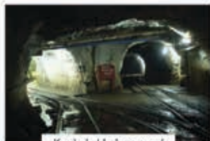
Konkola Underground Copper Mine, Zambia
