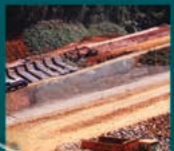
Drainage Channel - RENO MATTRESS® Ambalovy, Madagascar
