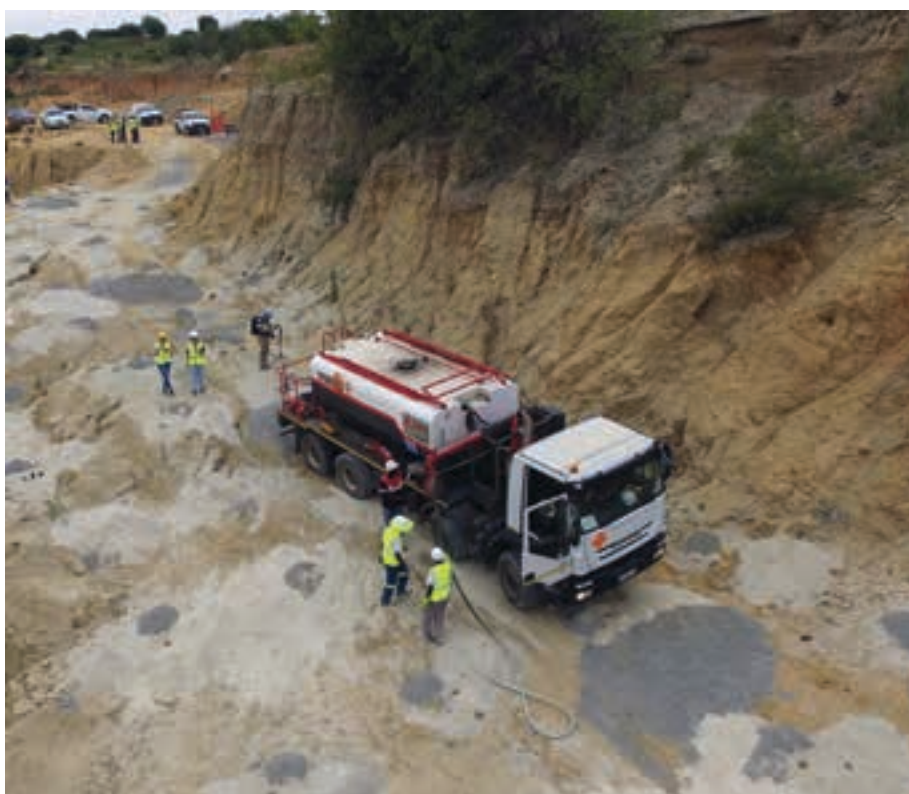
A view from a multi-copter of a blast in preparation.
