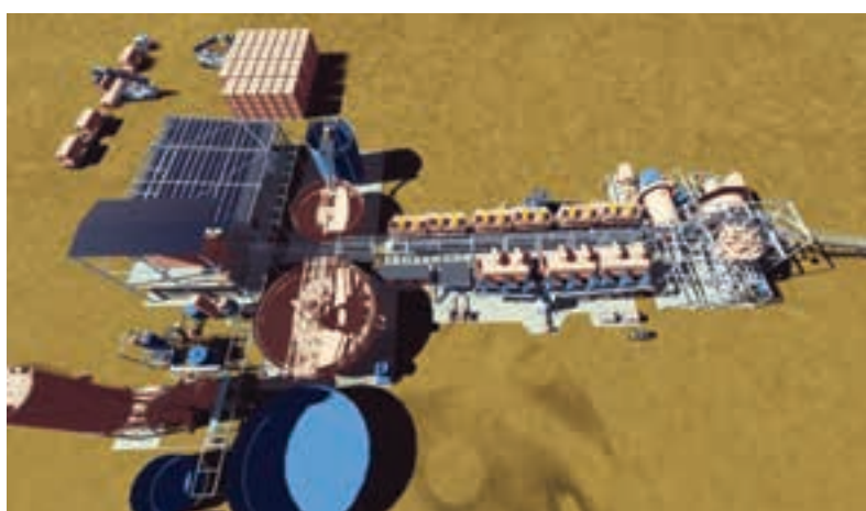
The 2 Mt/a sulphide flotation plant proposed for the T3 deposit.
