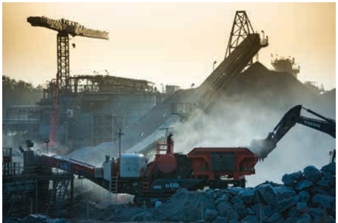
This recently commissioned Sandvik mobile crusher has boosted Asanko’s crushing capacity.
