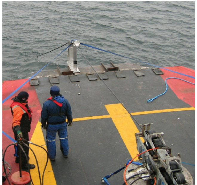
▲ Workers lay the cable on the bed of Lake Constance, Germany
