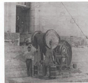
Two views of the original Otis Brothers steam internal geared freight elevator machine as it stands: view outside the monument. Machine lifted 12,500 pounds at 50 feet per minute, without a counterweight.
