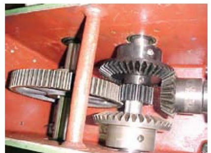
▲ Figure 5: Worn gears are replaced and a new motor installed
