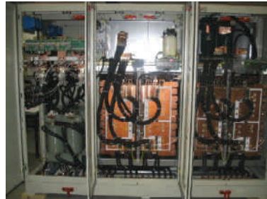
Figure 6: IGBT converter for a medium-frequency furnace
