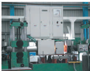
24" Pipe Mill And Annealing
