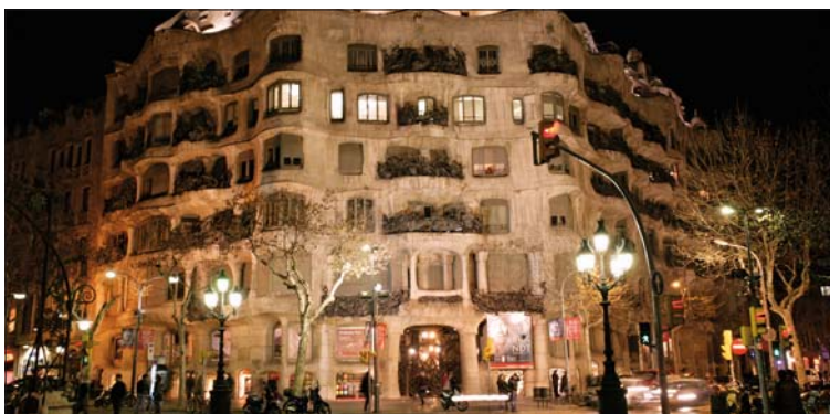
11 La Pedrera Page 117 • Apartment building or work of art? Both, when designed by Antoni Gaudí.
