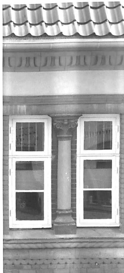
Facadedetalje mod gade
