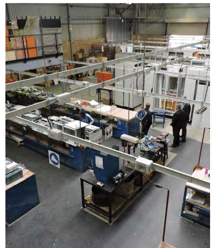
Low Voltage Switchboards is an independent panel assembler running production lines for the complete range of industrial control and automation equipment.
