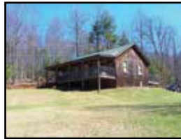
MLS 64175 - Galax - 1 BR , 1 BA, 900 sq. ft. Cabin, 40+ acres, stocked pond, abundant wildlife ATV trails throughout, newly installed well & septic, private but close to area amenities. $179,000
