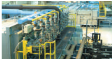
Can-Eng's continuous heat treatment system
