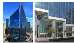
222 S 9TH STREET MINNEAPOLIS, MN
