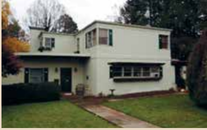
695728 339 COUNTRY CLUB ROAD - One of the more famous houses in Mount Airy, known as Dr. Renzo Sutter home, this strikingly modern house reflects the International style in its clean-cut, block, one and two story forms. Featuring LR w/ fp, dining, sun room overlooking gorgeous back yard, BR w/office, two bedrooms upstairs, 2 1/2 baths, kitchen with appliances, plus lots of character and natural light with corner windows. Sitting right at Mount Airy Country Club!.....$160,000
