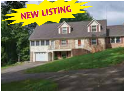
627 Knollwood Drive (Mt. Airy Country Club)- "Just How Much Home Do You Need?" 3 or 4 Bedrooms, 3 Full Baths (1 Has Steam Shower) Kitchen w/ Appliances, Dining Room, Large LR w/ Fireplace w/ Gas Logs, Huge Sunroom w/ Gas FP, Office, Laundry Room, Attached Garage; Play Room; Decks and Porches for Relaxing; Double Paved Driveways w/ Circle Drive; Complete New Roof! Security System, Heat Pump/ Central Air; 2 Lots totally 1.38 AC. This home offers so much for a Family!.....$169,900
