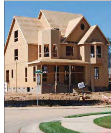
Residential construction at the Savannah subdivision.
