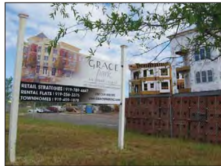
Mixed use construction (rental flats over retail) at Grace Park.
