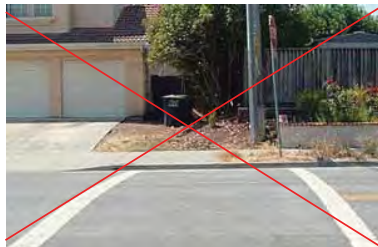
Curb ramps should be included at all intersections and pedestrian crossings, and be directed towards crosswalks to improve safety and connectivity.
