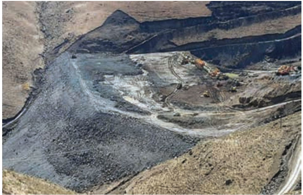
Toe of the new slimes dam wall (September 2015).
