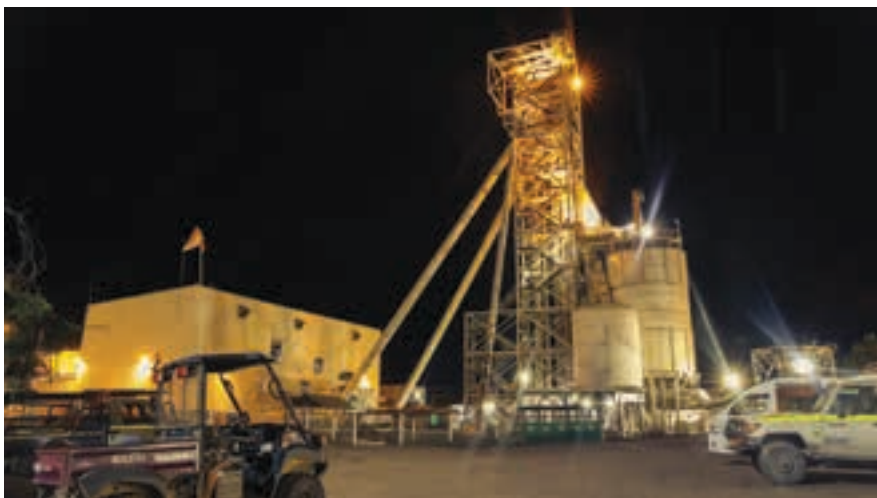
Bulyanhulu – which was commissioned in 2001 – is an underground mine with shaft access, which is transitioning to long-hole and drift and fill as its principal mining methods (photo: Acacia).
