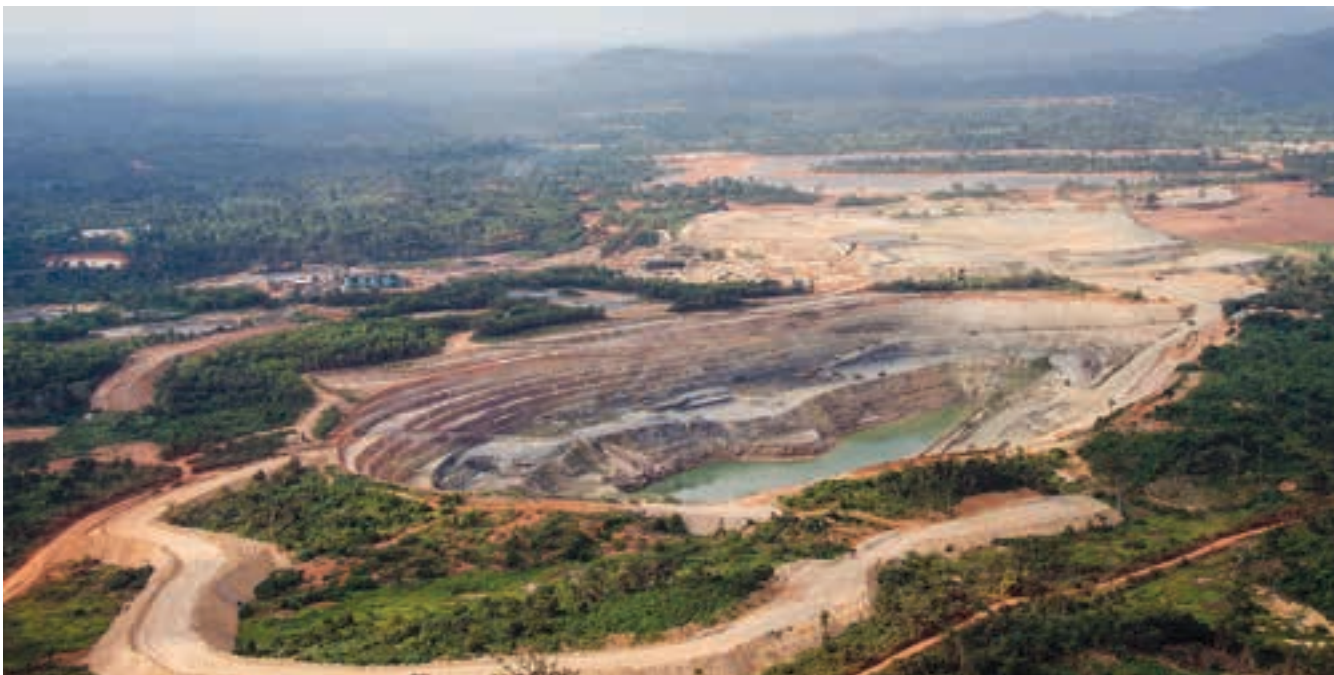
The Asanko site showing the main Nkran pit. Dewatering of the pit is well advanced and should be complete by November (photo: Asanko Gold).
