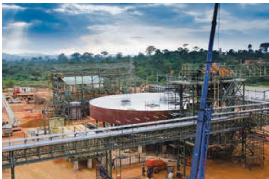
Pre-leach thickener under construction at Asanko (photo: Asanko Gold).
