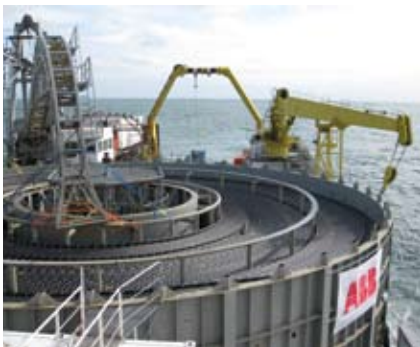
○ Cable loaded onto a turntable, onboard a cable-laying vessel
