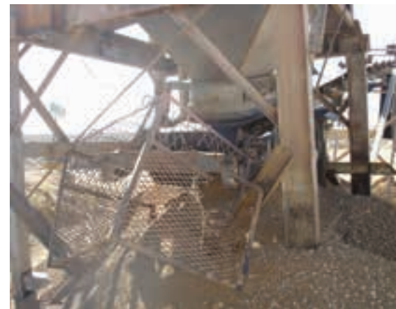
In small sand and gravel quarry operations, which are less profitable, and where conveyors are built and modified without professional design, conveyors may well be inadequately guarded (courtesy Marius van Deventer).
