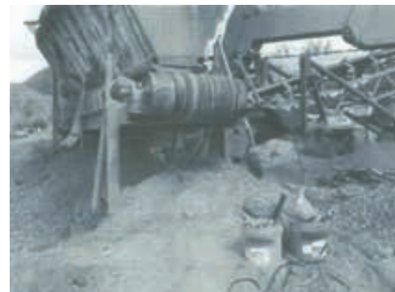
Figure 7: Unguarded pulley and conveyor [4]. Picture indicates a similar conveyor, completely unguarded, and again with considerable material build-up. In addition, in this instance, poor maintenance is clearly visible, including the poor alignment of the head pulley and resultant poor tracking of the belt.
