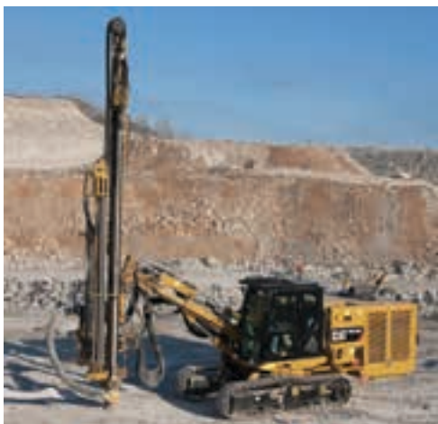
The Cat MD5150C top hammer drill at Tower Rock.
