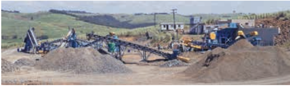
The Pilot modular custom-built plant has now increased Umhlali Quarry's output of road stone aggregate.
