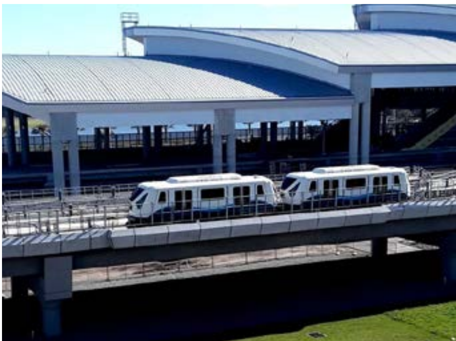
The new South APM connecting the Main Terminal to the South ITF
