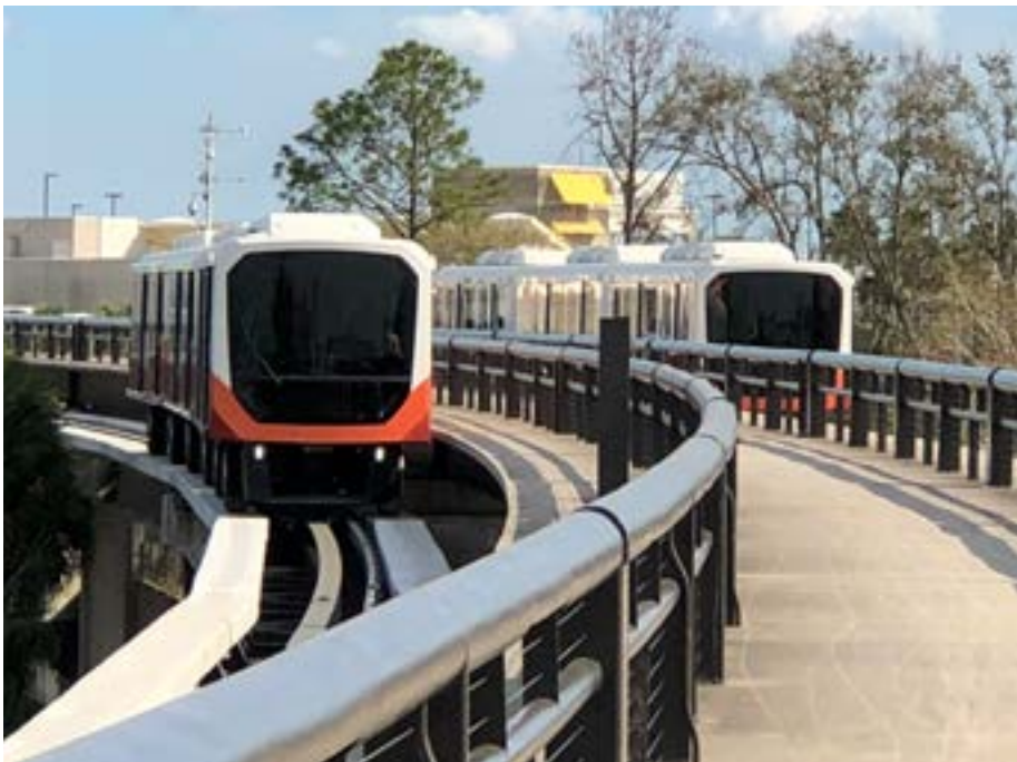
The new Orlando Airport Airside 1 (2300 & 2400) APMs
