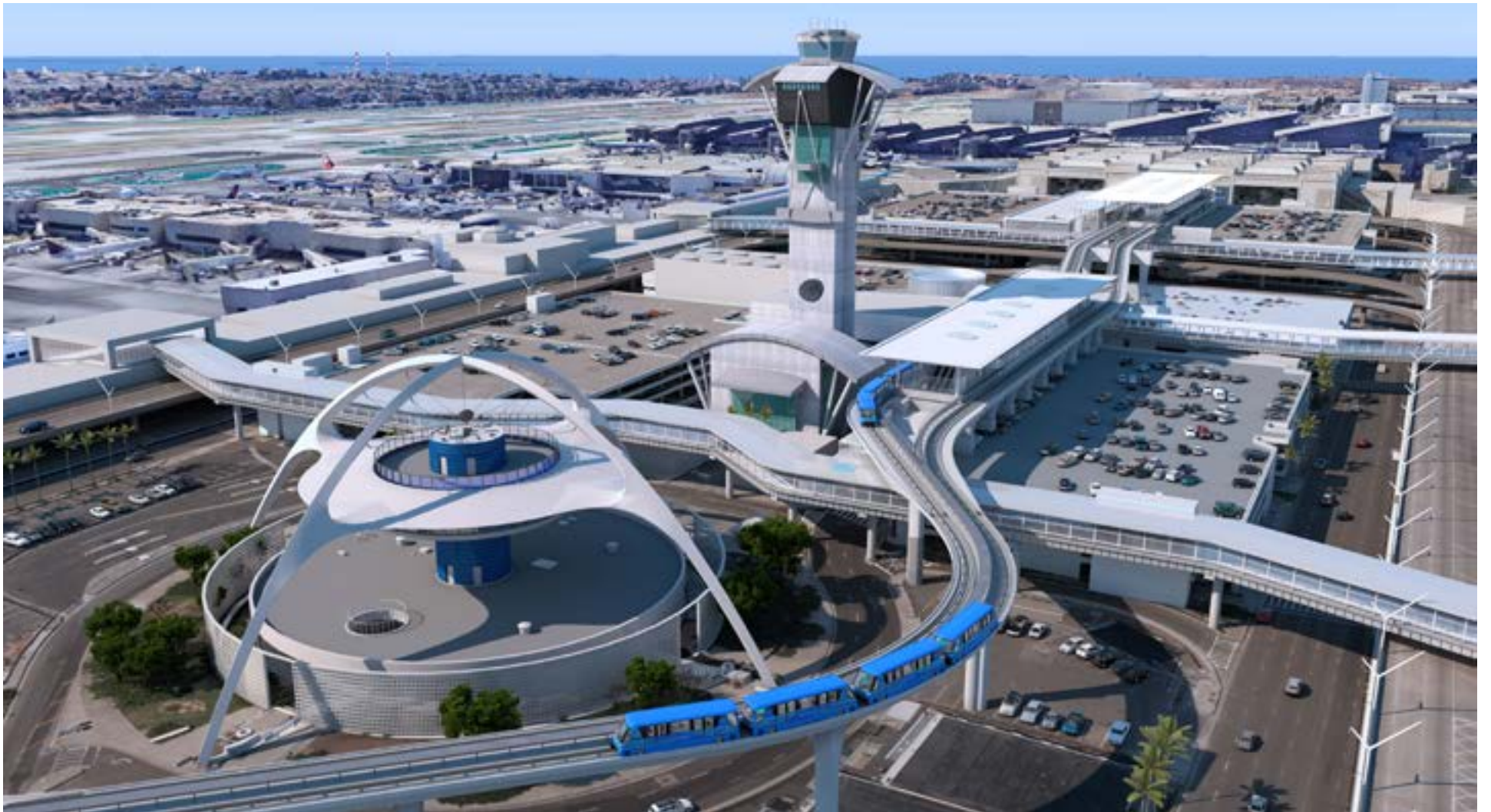
Aerial of Automated People Mover Train Image credit: LAWA
