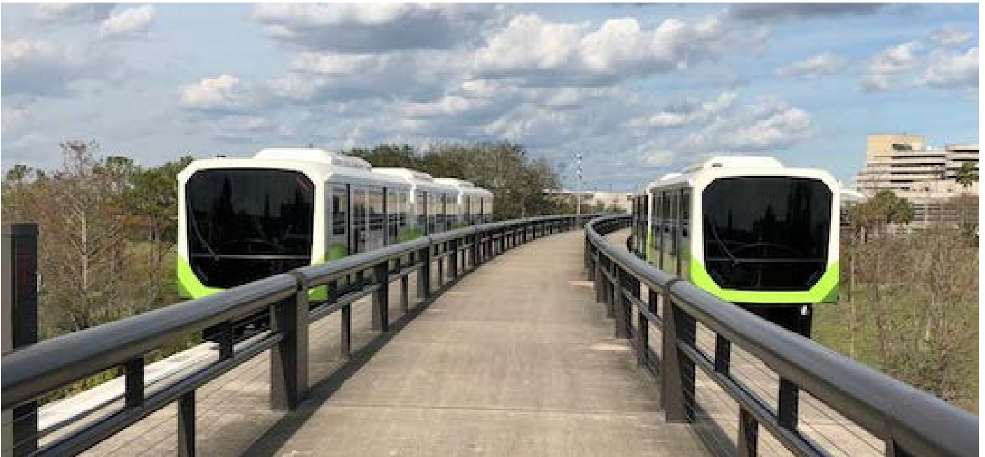
The new Orlando Airport Airside 3 (2100 & 2200) APMs
