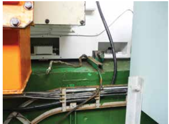
Figure 7: Not the way to earth a motor.
