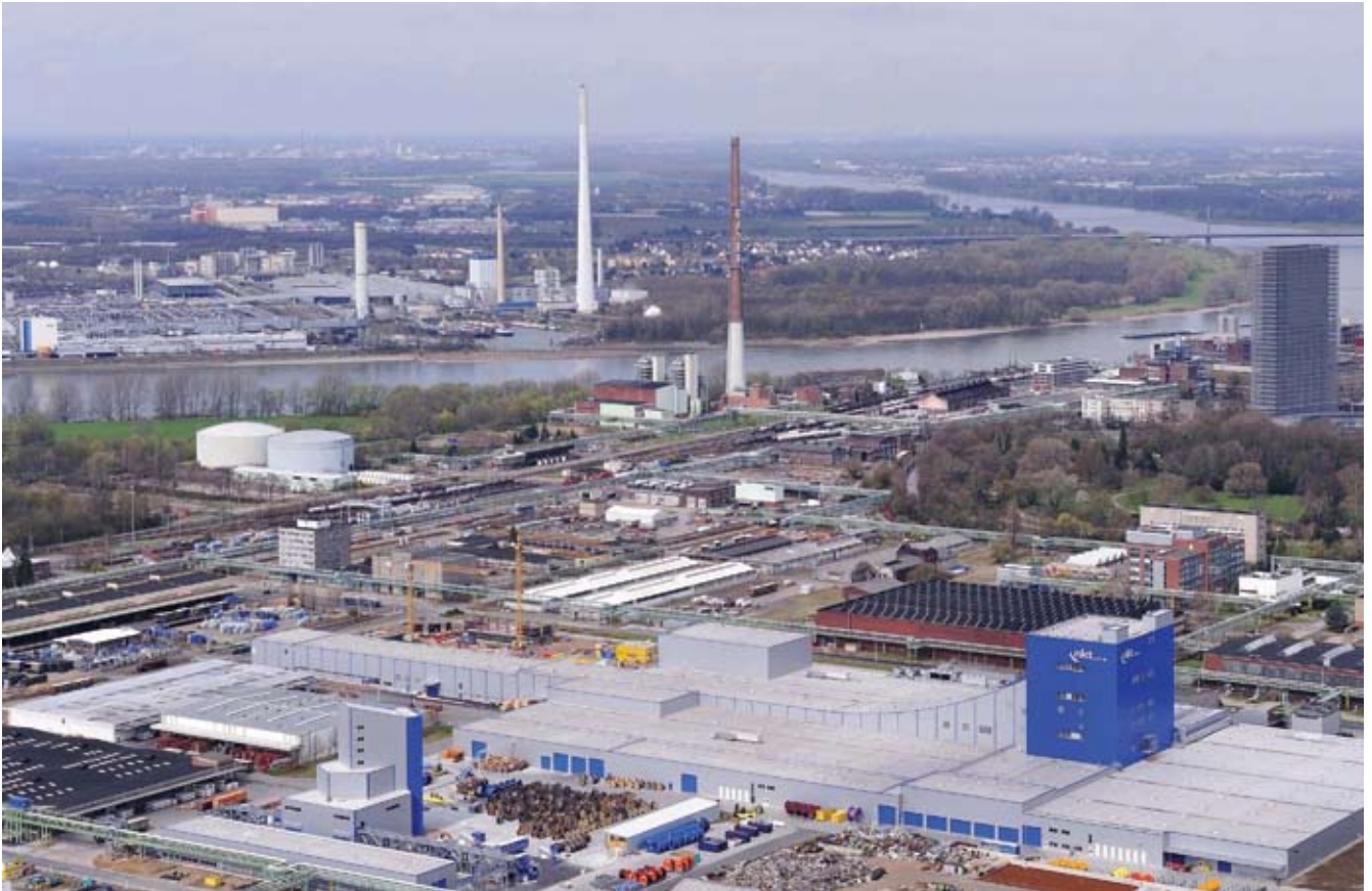
▲ The new nkt factory in Germany
