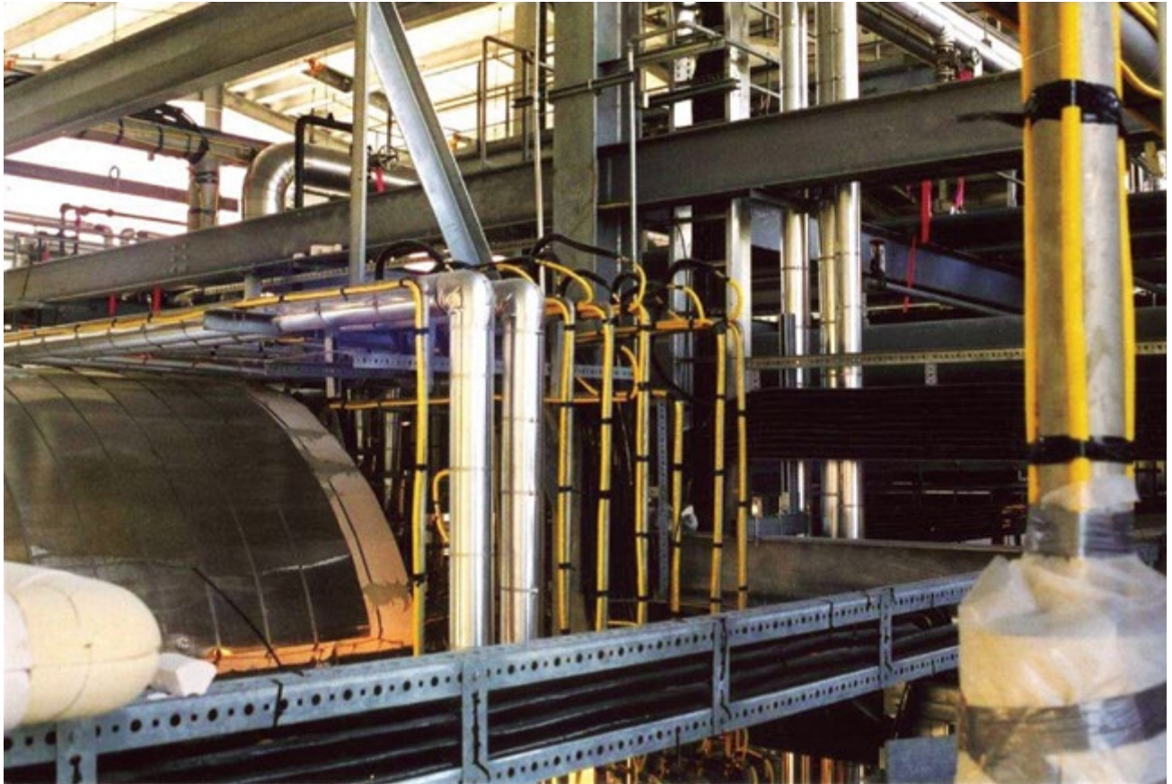
Figure 2: 'Safe Trace' installation.
