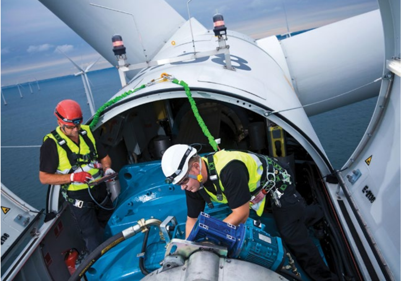
Figure 2: Routine maintenance performed up-tower (courtesy Siemens).
