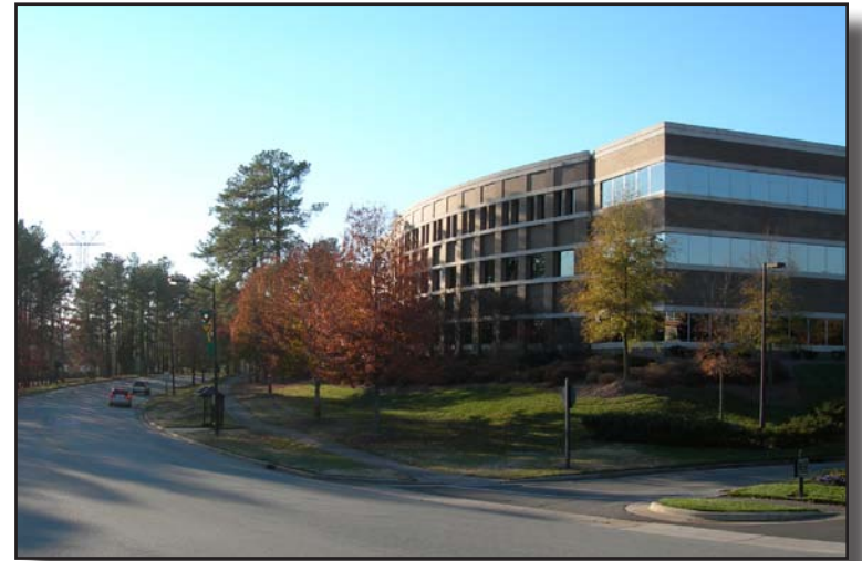
Local office building.
