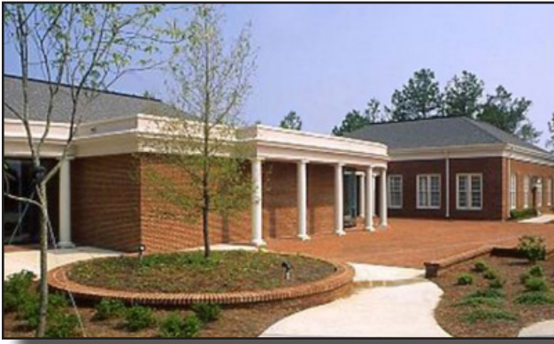
The Morrisville Town Hall is a good example of a landmark building that stands apart from its surroundings, but is compatible with neighboring uses.
