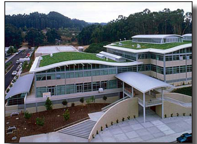
Office buildings can reduce the loss of green space and increase energy efficiency by incorporating green building design techniques. In this example, the roof of the building is covered with native grasses and wildflowers, which provides habitat for plants and animals, slows water run-off into local storm drains, and provides extra insulation to help heat and cool the building.
