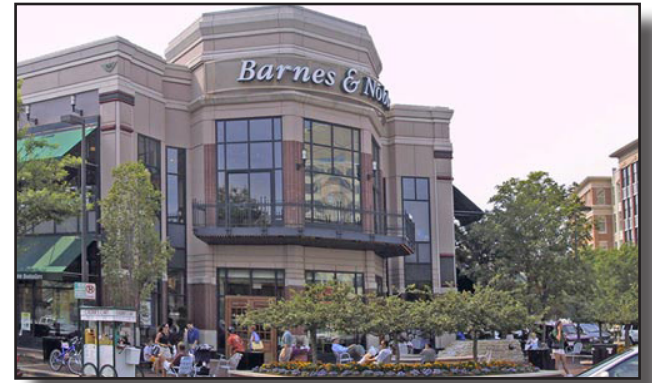
This fountain and plaza located at the entrance of a large retail establishment act as a central meeting and gathering place.
