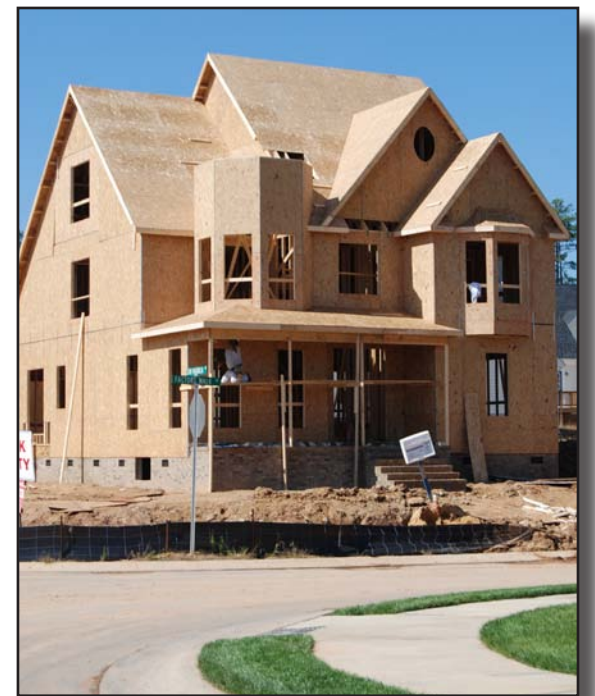
Residential construction at the Savannah subdivision.
