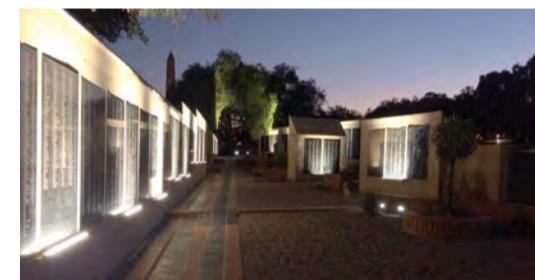
Linear LED luminaires light up the façade of the walls in the Garden of Remembrance.
