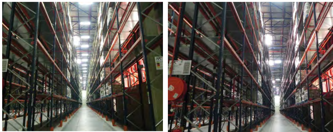
Before and after images show how Magnet's wireless Lite-C system controls lighting by ensuring lighting is turned off when aisles of this warehouse are not occupied.
