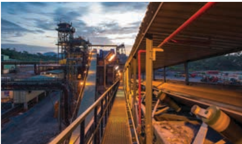
Another view of the processing plant site. The current capacity of the processing facilities is 3 Mt/a.
