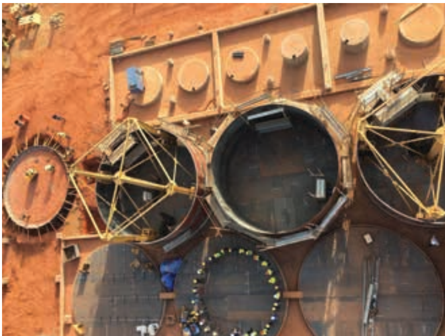
CIL tank construction at Yanfolila earlier this year (photo: Hummingbird).
