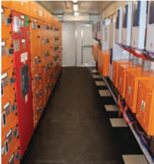
A major benefit of containerised substations is that they are fully equipped and assembled at the manufacturer's premises.
