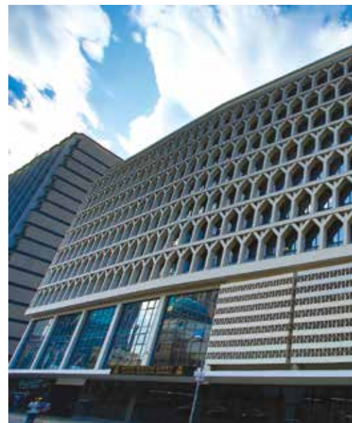
TAL supplied adhesives for the installation to refurbish the Innes Chambers office building.
