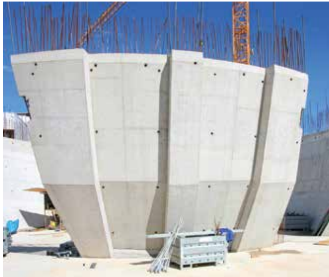
ABOVE: All of the assembly work for these highly sophisticated formwork panels is completed at the Doka Pre-assembly Service. BELOW: Fine adjustments are accomplished by using top-mounted forming boxes. Photos: Doka
