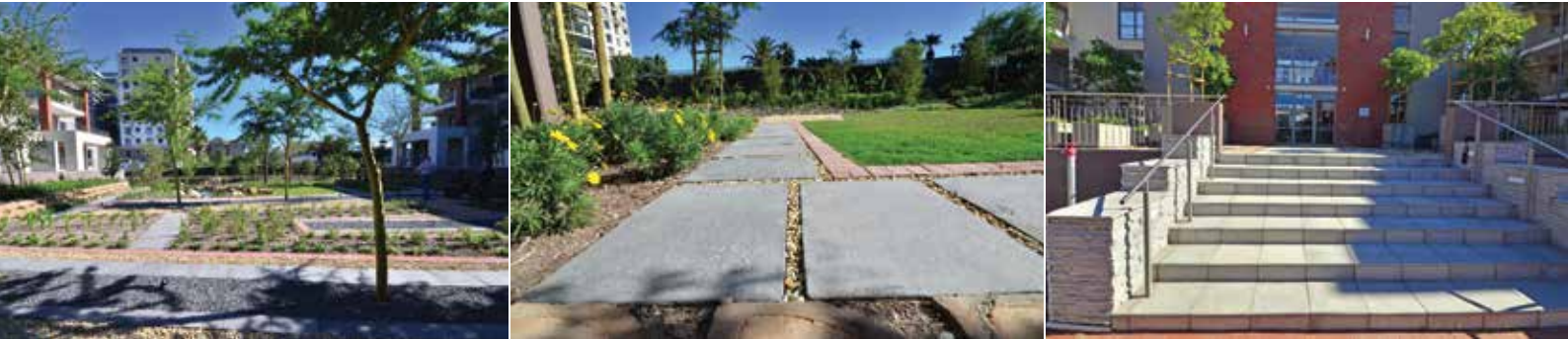
PHOTOS FROM LEFT: One of the elevated courtyards where Revelstone's Ravine and Random Edge pavers were used to delineate and embellish gravel sections; Kent Random Edge pavers interspersed between lawn and flower beds create an attractive and durable path; and a combination of Revelstone paving, tiling and cladding products make for an imposing staircase.
