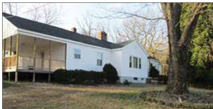
535 ALLRED MILL RD, MT. AIRY, NC; 2-3 Bedroom with dining area, Kitchen new tile countertops, Large Den with built in shelves, LR with FP, office/bedroom, laundry room , 2 baths with all new tile work, all new vinyl siding, New roof, New vinyl windows, double detached garage, 12 x 12 storage building, over 2 acres of land, convenient location , over 1600 + SF . $134900 Call for an appointment today – 336-789-1365
