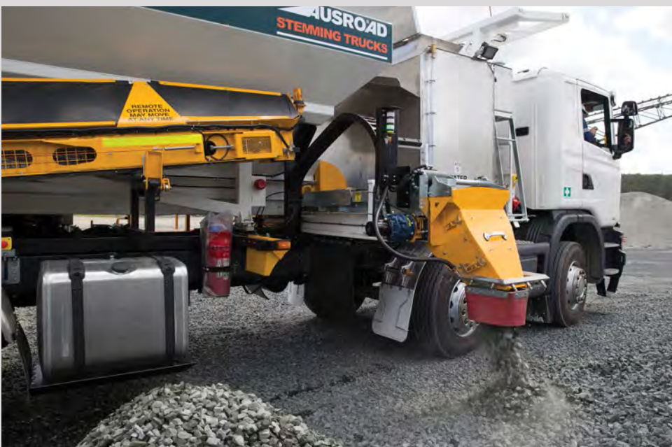
Aggregate being dispensed.
