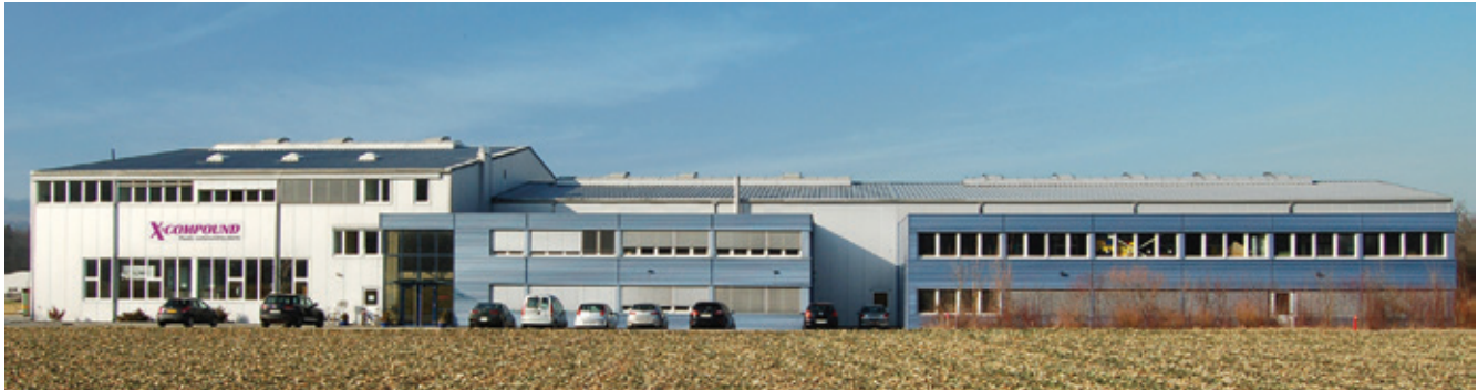
▲ The X-Compound site at Kaisten, Switzerland
