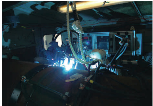
CRC-Evans offer a range of automatic welding systems for land and offshore pipeline construction
