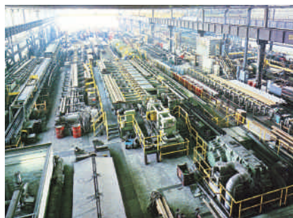
Ⓜ Hagering's complete 1,600kN tube drawing plant including handling and swaging machine
