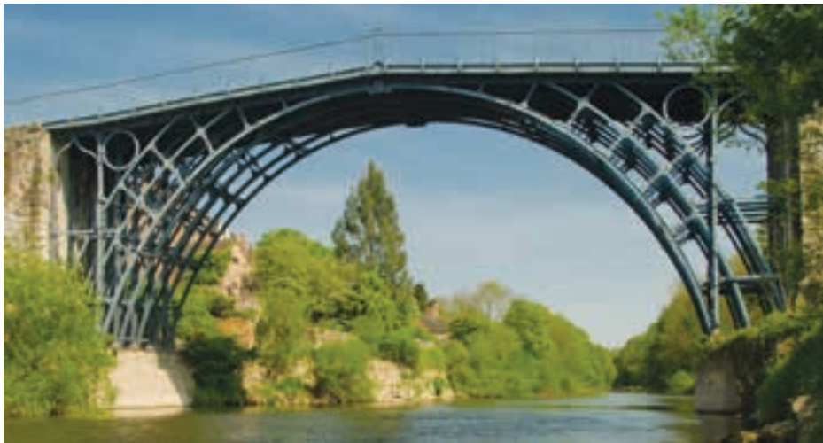
The first iron bridge was opened on New Year's Day 1781 and still stands in the town of Ironbridge, west of Birmingham.
